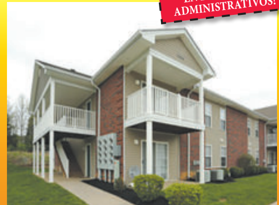
AUSTIN PARK APARTMENTS 201 Pheasant Ave. Louisville, KY 40118 502-368-9991 www.Austinpark-apts.com 1, 2 & 3 Bedroom Apartments
