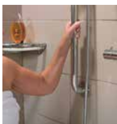
Riser safety grab bar
