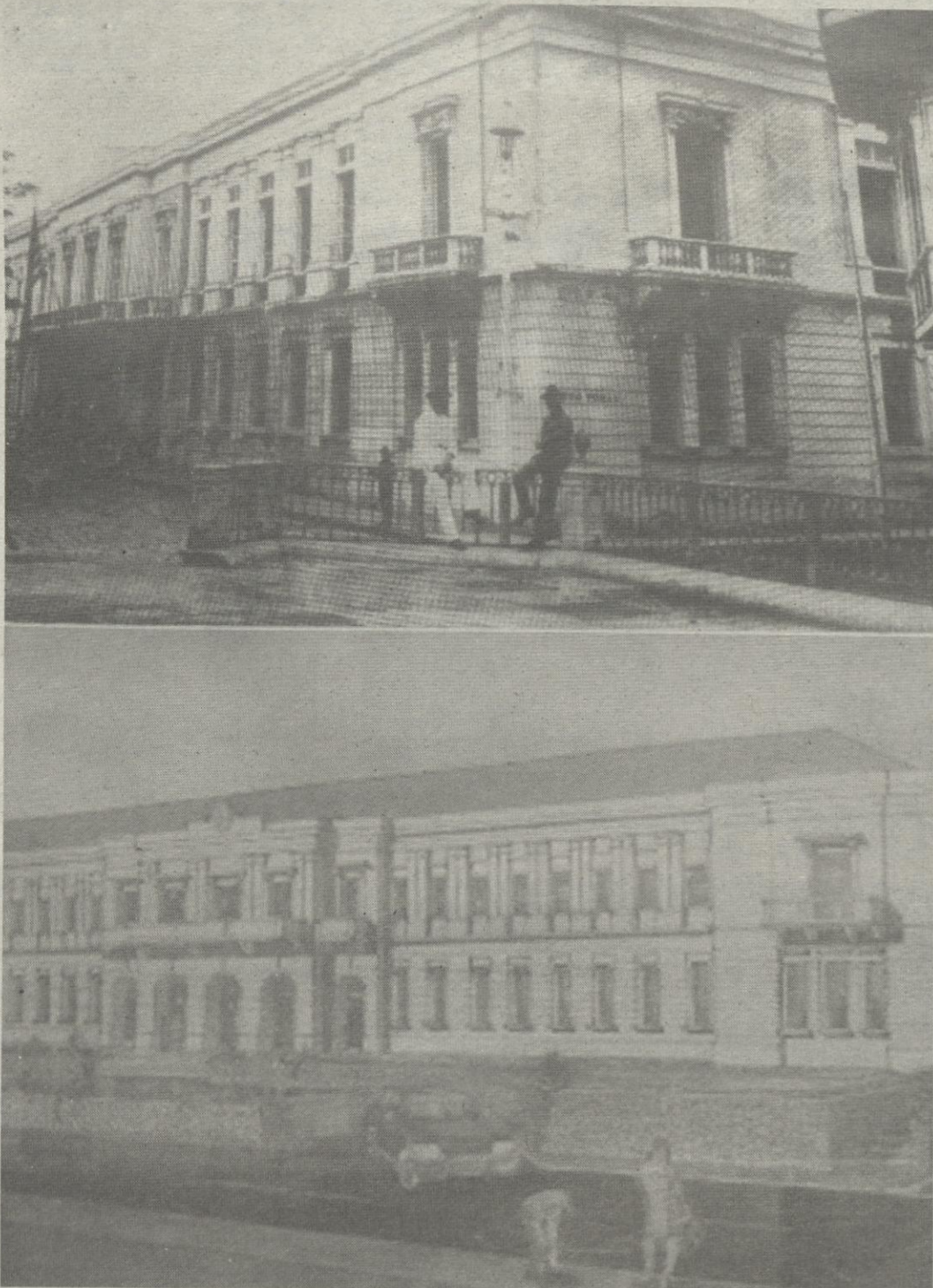
Then and now. The Ayuntamiento of the Spanish era (above) serves as the inspiration for the new Administration Building (perspective below). Photos by Jasmyn Sade and Aubrey Farillon
