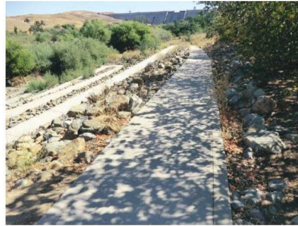
Figure 3.2: Class I Shared-Use Path: a path in separate right-of-way; typically makes use of scenic resources
