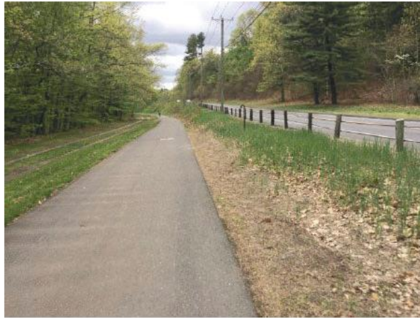
Figure 3.1: Sidepath: a path within a road right-of-way; direct and convenient but potentially less scenic
