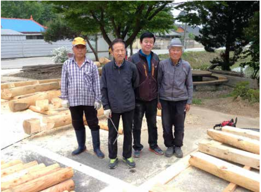
The local crew at Maeyo-ri working on the new jeong-ja.
