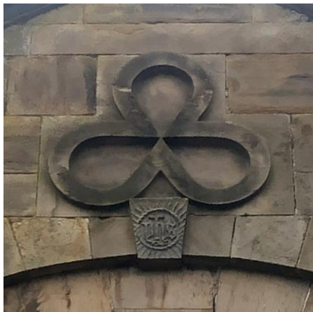
[Figure 22] The trefoil and IHS keystone above the entrance. Photograph by author.
