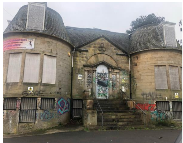
[Figure 2] Gracemount Mansion, Front Facade, 2024. Photograph by author.
