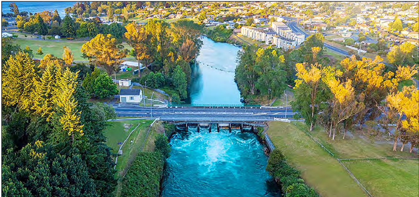
An aerial view of the Control Gates bridge in Taupō.
