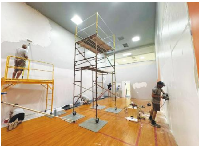
ALL HANDS ON DECK: The renovation work is well underway.
