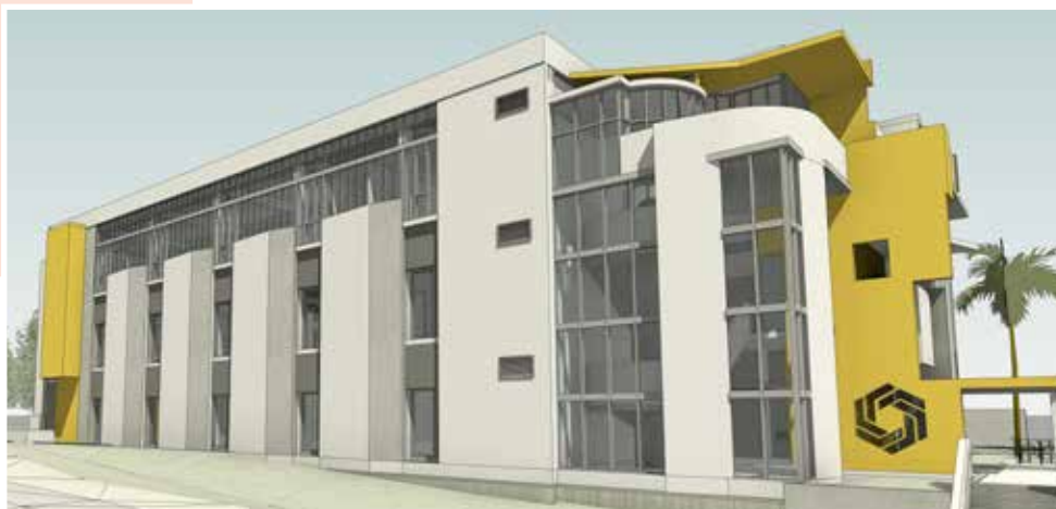
The Forward Center, a second building construction at Science City, will be ready at early 2023.
