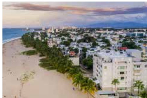
Carrion Court Villas Type: Ground Up Townhome Size: 50,000 GSF Status: Portfolio Asset Under Construction
