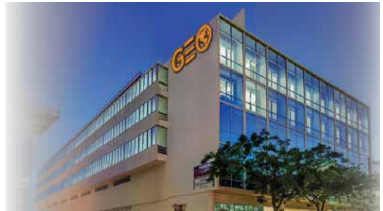
GEO Tax's headquarter's at 1064 Ponce de León Ave. in Santurce, Puerto Rico.
