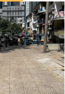
Pedestrian path was unable to be used due to vehicle illegal parking
