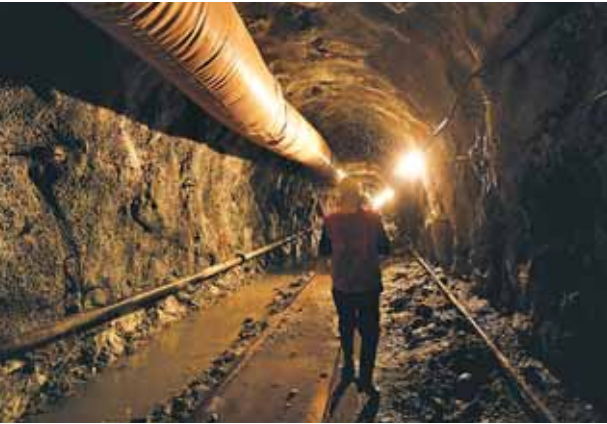
Tunnel of Melamchi Khanepani Project, Nepal.
