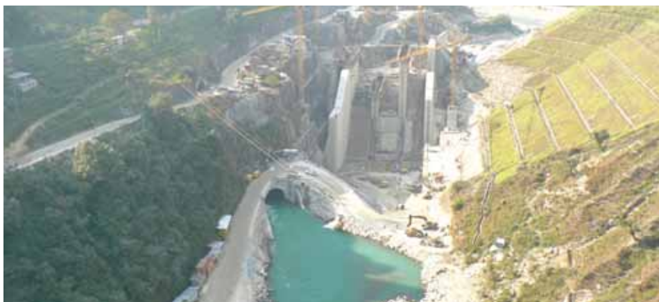
Middle Marsyangdi hydroelectric Nepal.
