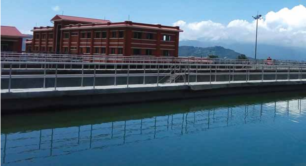
Under Construction Melamchi Khanepani Project, Nepal.
