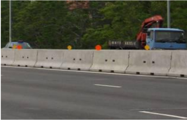
Fig. 5.16 New Jersey Barrier
