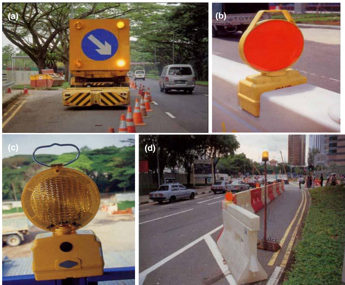
Fig. 5.22 Types of Lighting Devices (a) Truck Mounted attenuator; (b) Warning Lights; (c) Flashing Warning Beacons; (d) Rotating Amber Light
