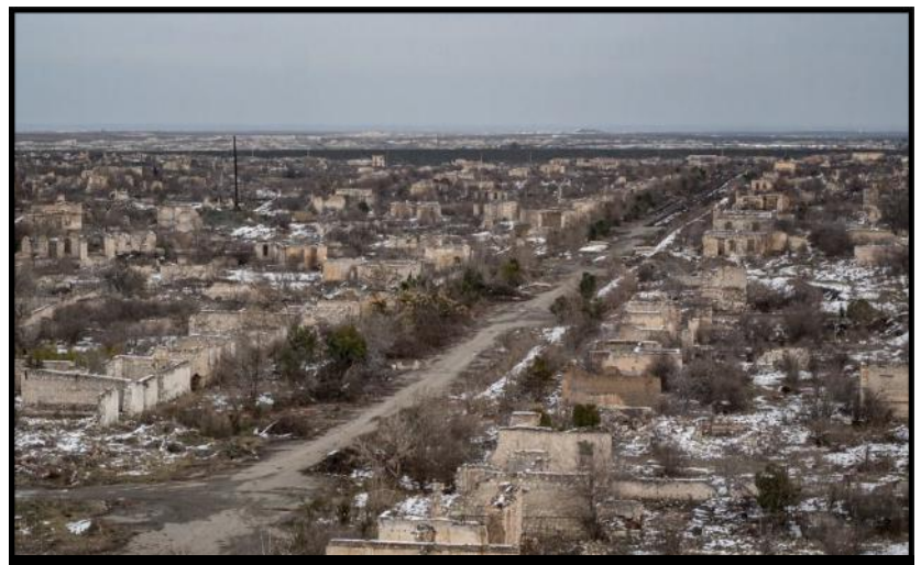
Total destruction of the town of Agdam
