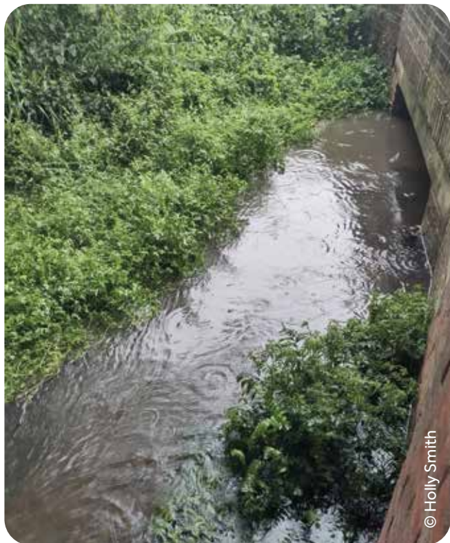
Germain Street Bridge
