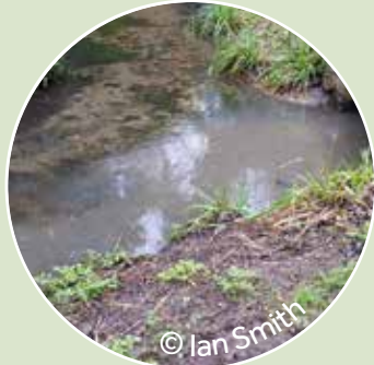
Vale Brook Culvert
