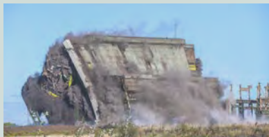
Figure 11. The former Redcar Coke Ovens were demolished with 175kg of explosives. On the same day, the air quality monitor in nearby Dormanstown for PM10 spiked to 50 micrograms per cubic metre from 7.5 an hour before (Mazza, 2022).
