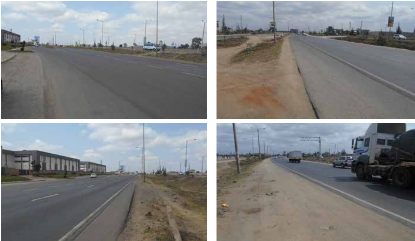
Picture: Part of Machakos Nairobi border road section
