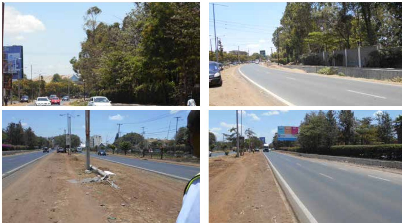
Picture: Part of Sunshine School road section
