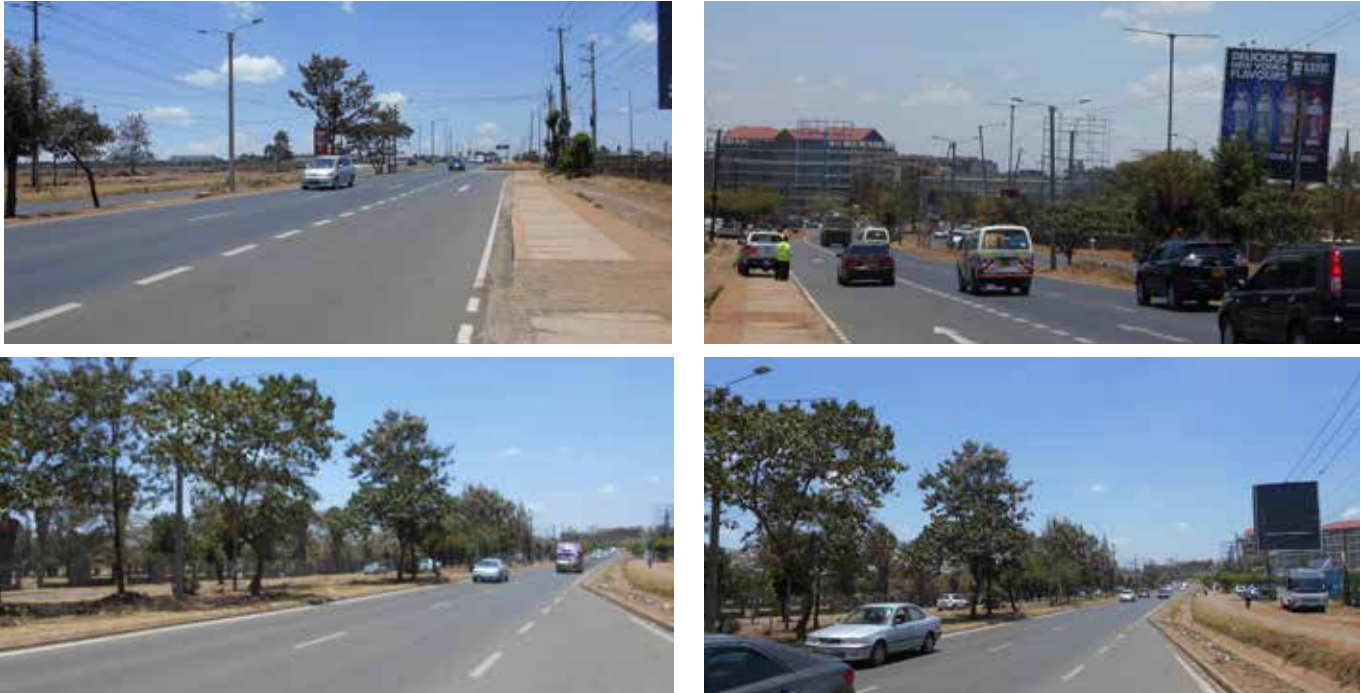
Picture: Part of Langata Road Southern Bypass Interchange road section
