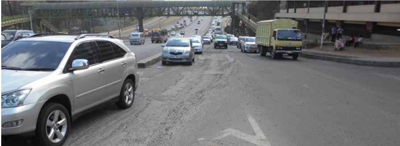
Picture: Part of Kwa Kirima road section
