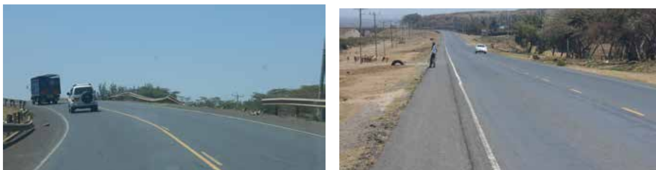
Picture: Part of Oasis Area road section
