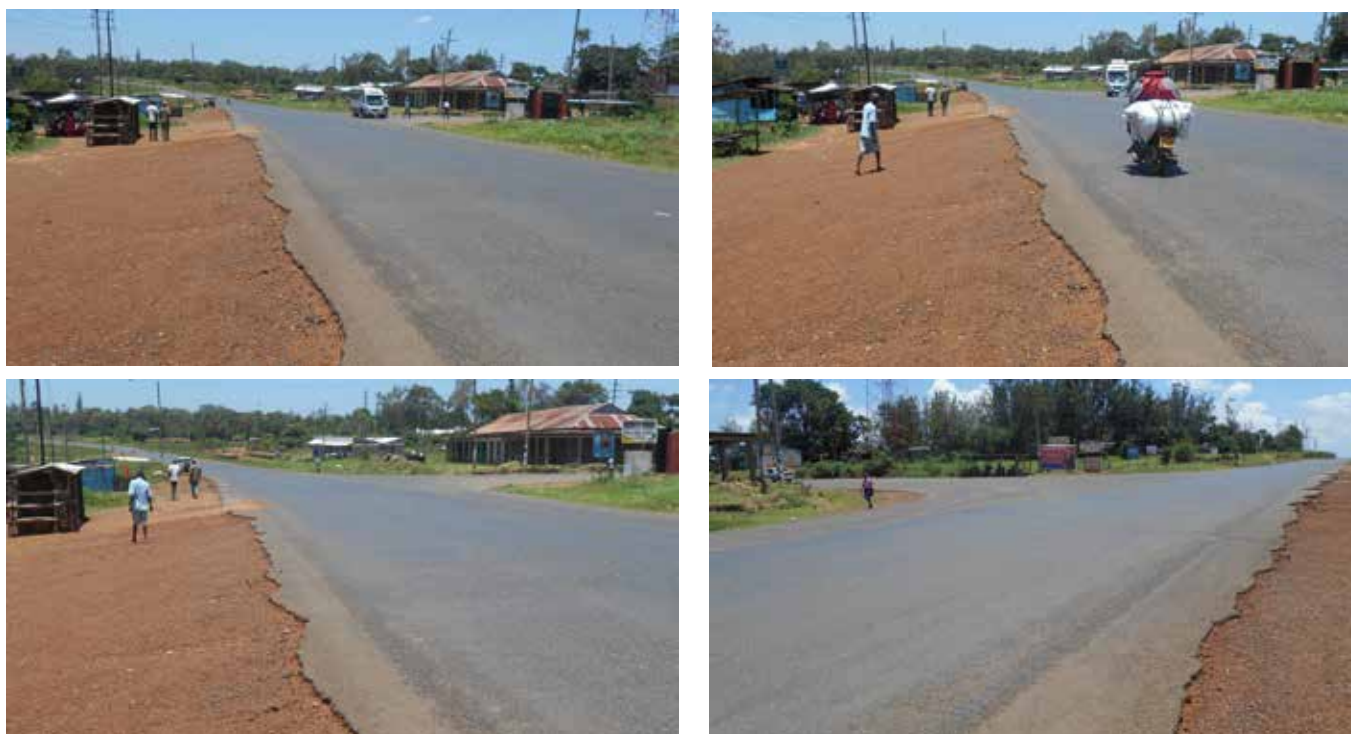
Picture: Part of Rangala junction road section
