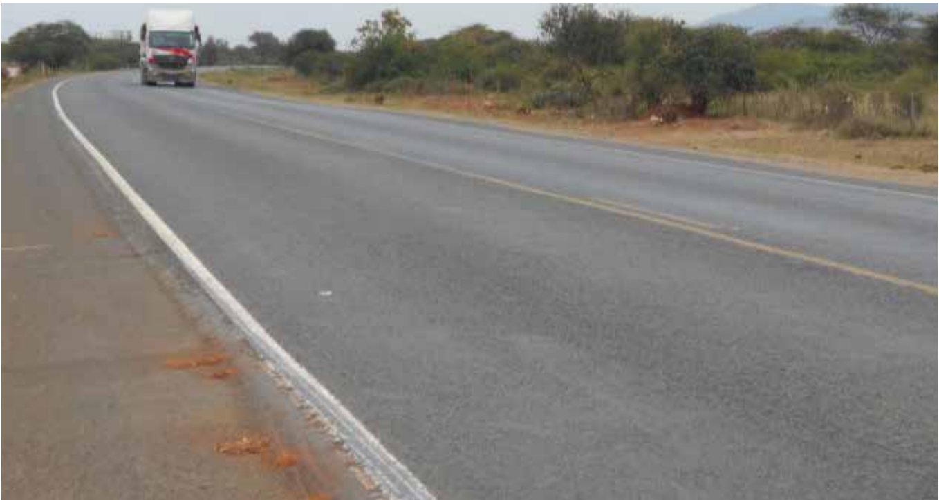
Picture: Part of Kwa Msomba road section
