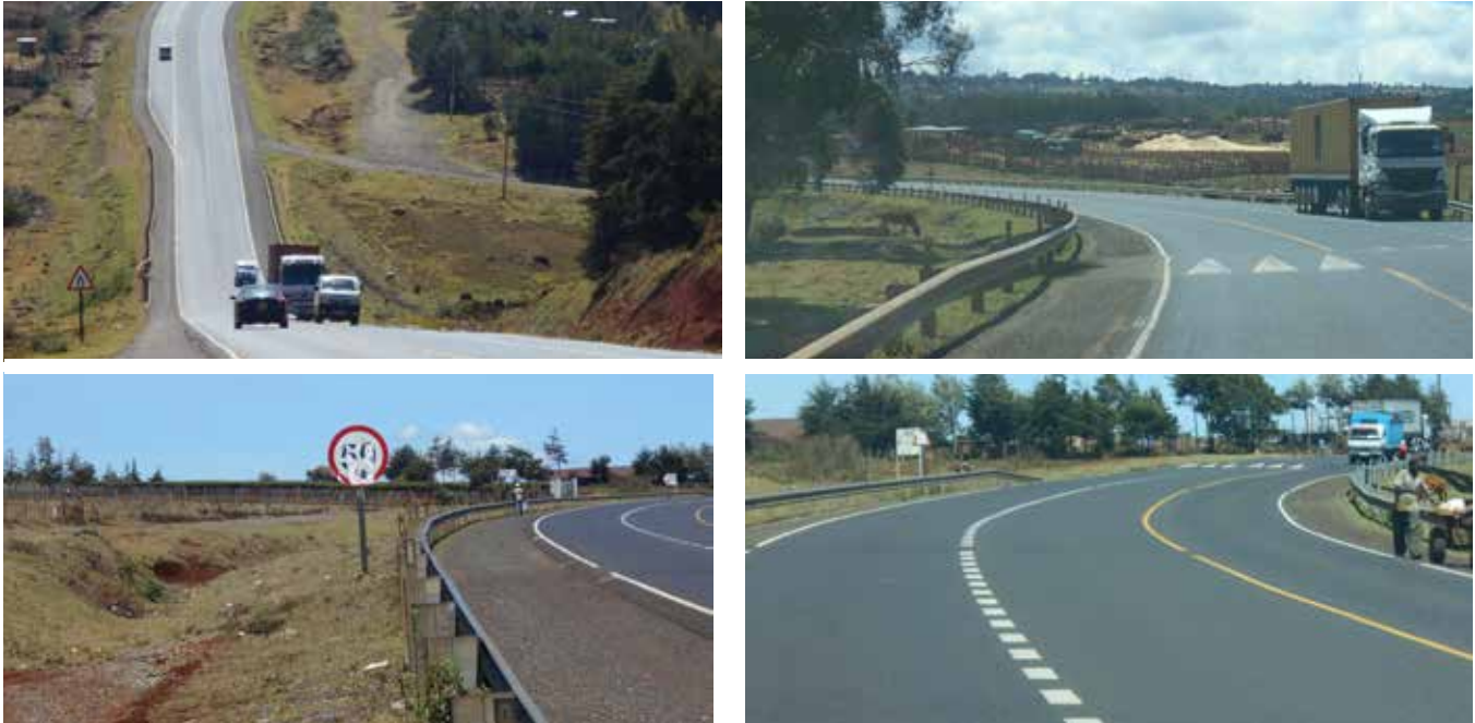
Picture: Part of Matharu - Chirchir road section
