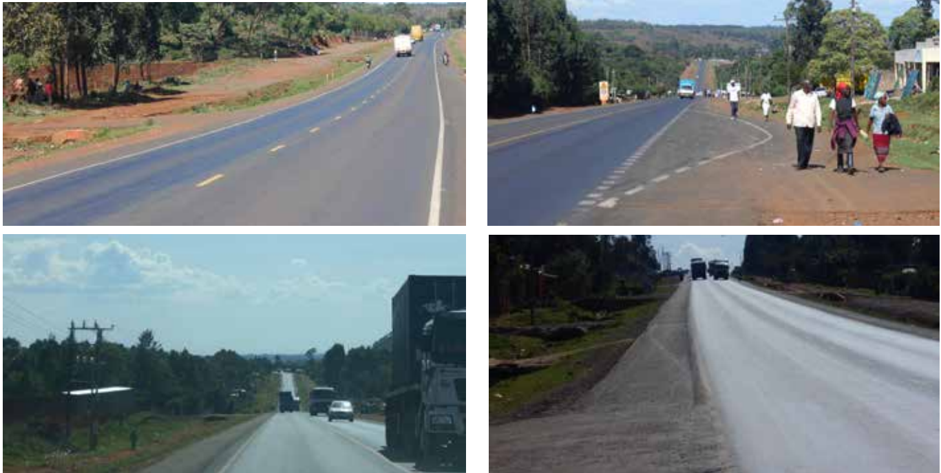
Picture: Part of Mwamba Area road section
