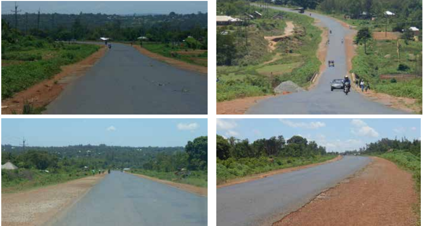
Picture: Part of Naam Nzoia road section
