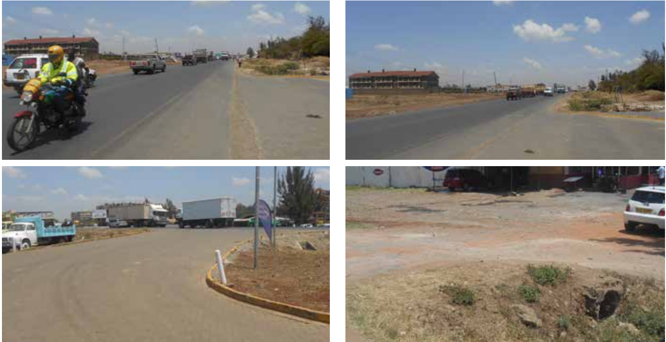
Picture: Part of Delta Petrol Station road section
