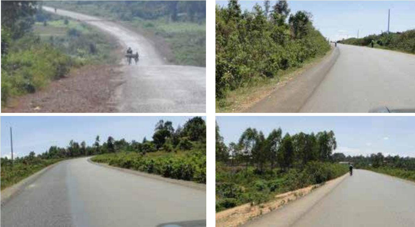
Picture: Part of Dudi road section
