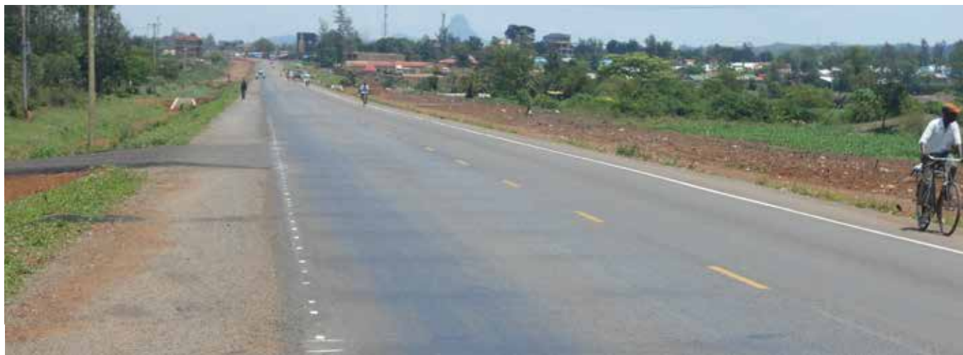
Picture: Part of Ikapalok - Malaba road section
