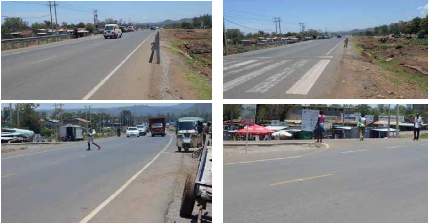
Picture: Part of Otonglo Area road section
