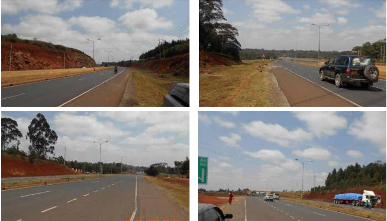
Picture: Part of Southern Bypass near Dagoretti road section
