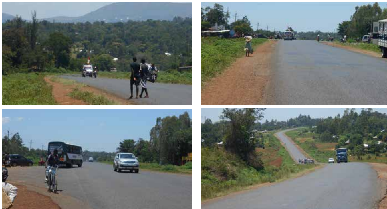
Picture: Part of Got Nanga road section
