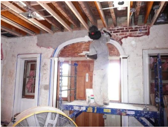
Plaster work in central room, 2011. FCPA photo.
