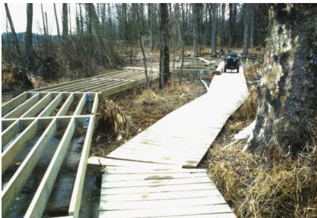
New boardwalk being constructed next to original boardwalk, February 1993.FCPA photo.
