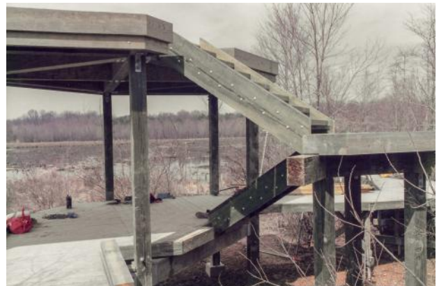
New observation platform under construction, 1993 . Photo by volunteer Stan Russell.
