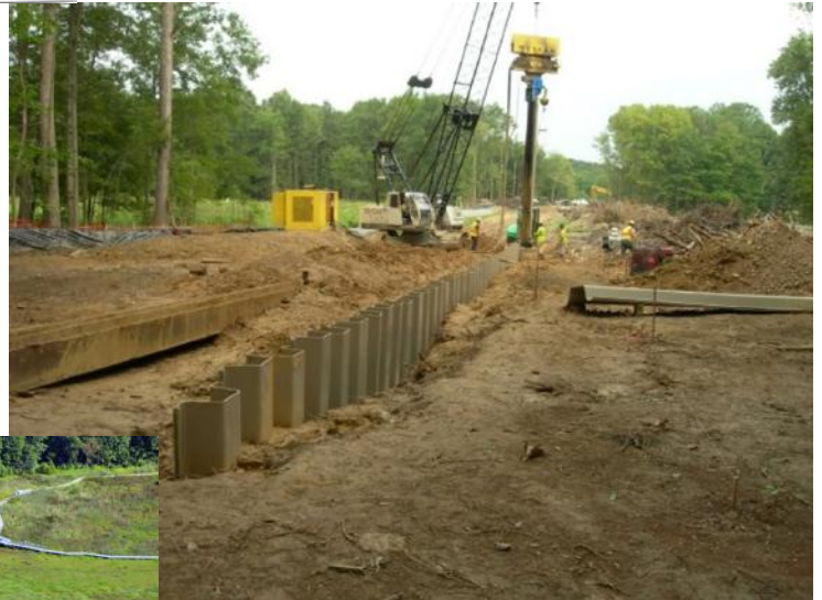
Installation of Berm Core, August 2013. FCPA photo.
