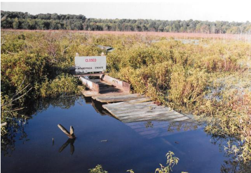
High water levels flooded the original boardwalk. HMP staff closed sections beginning in 1991, with the entire boardwalk closed on October 28, 1992, Photo by volunteer Stan Russell.
