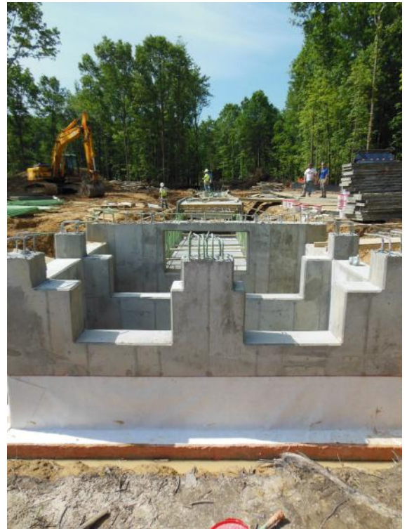
Installation of Spillway, June 2013. FCPA photo.
