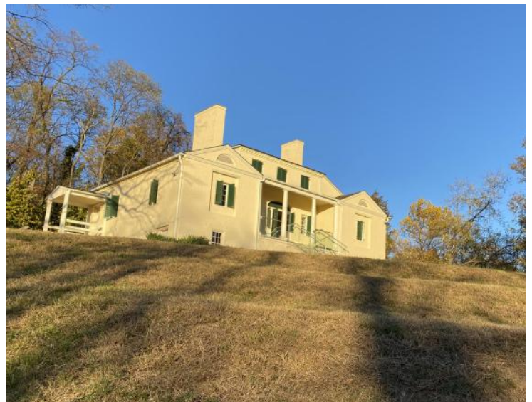
Restored Historic Huntley, south front. Photo by Carolyn Gamble.
