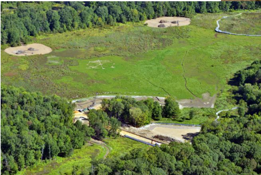
Overview of completed work, showing habitat pools, 2013. FCPA photo.
