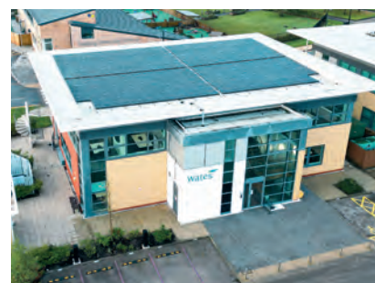
Smartspace recently upgraded its Warrington office from an EPC C rating to EPC A+, with over 92 per cent of waste diverted from landfill. The office now has 64 kWp photovoltaic array.
