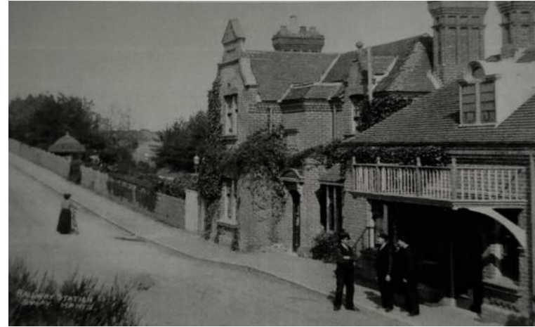
Sway Railway Station
