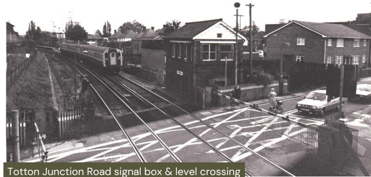
Totton Junction Road signal box & level crossing
