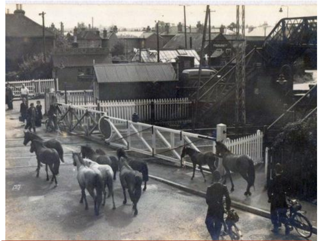
Ponies on Junction Rd Level Crossing, Totton Historical Society
