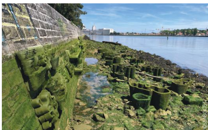
Figure 1: Tidal pools can be attached to vertical walls, placed at the base of breakwater or quay walls
