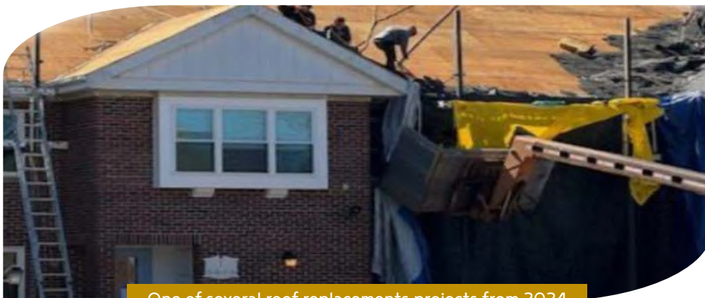
One of several roof replacements projects from 2024
