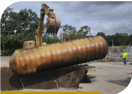
Removal of old fuel tanks at DPW Garage (70 Elm St.)
