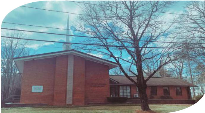
COMMUNITY CENTER AT 76 MAIN STREET
