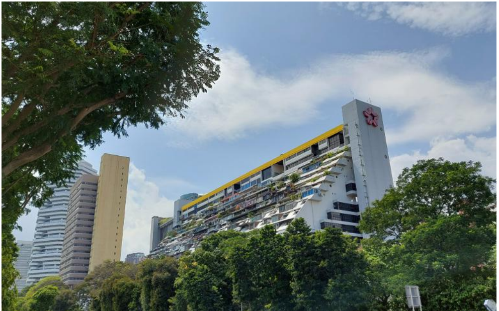
Figure 46. Golden Mile Complex marks an important mile stone in the conservation of a significant modern heritage buildings in Singapore, a decision based on economic viability and place memory. All images are from the author unless otherwise stated.
