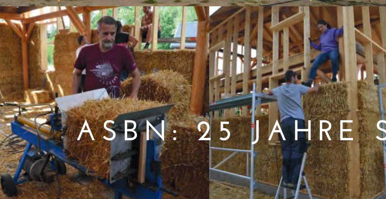
Strohballenhaus in CUT-Technik, Laxa, SE (Details: strohnatur.at). Compression of the straw bales with a converted wood splitter (below)
