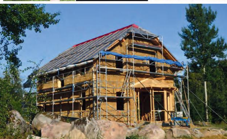
Strohballenhaus in CUT-Technik, Laxa, SE (Details: strohnatur.at). Compression of the straw bales with a converted wood splitter (below)
