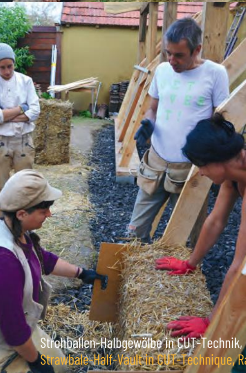
Strawbale-Wrapping in Gmünd (Details: strohnatur.at ).
