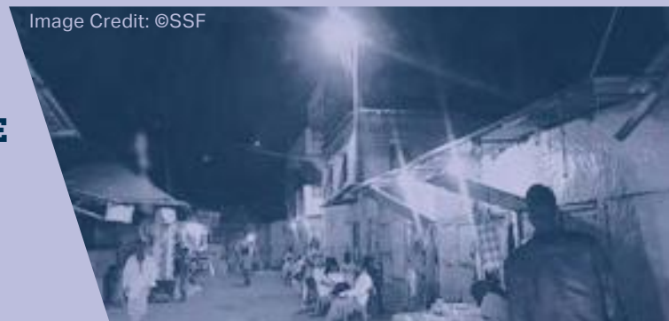
Residents in Galdogob carry out their business at night following installation of solar lights by SSF.
