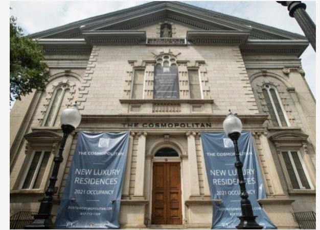
The Cosmopolitan — the former Church of Immaculate Conception built in 1850 — has been reimagined as 63 luxury condominiums in Boston's historic South End neighborhood. Source: Preservation of Affordable Housing
