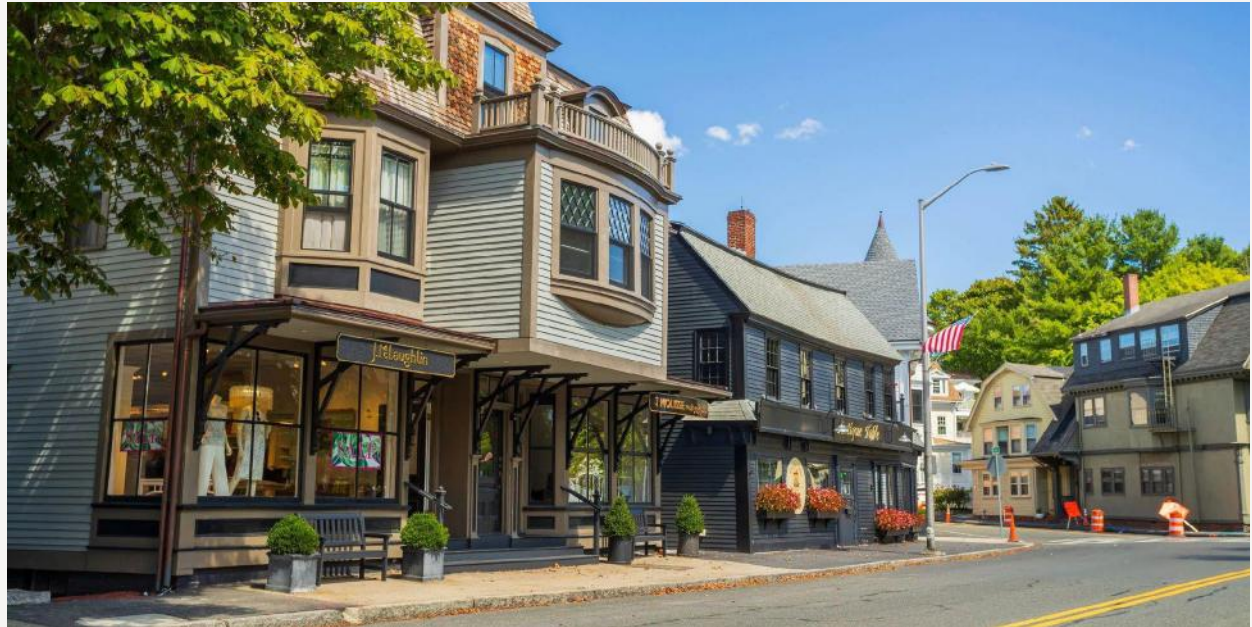
This section of Manchester's downtown does not comply with current zoning. Source: class photography
