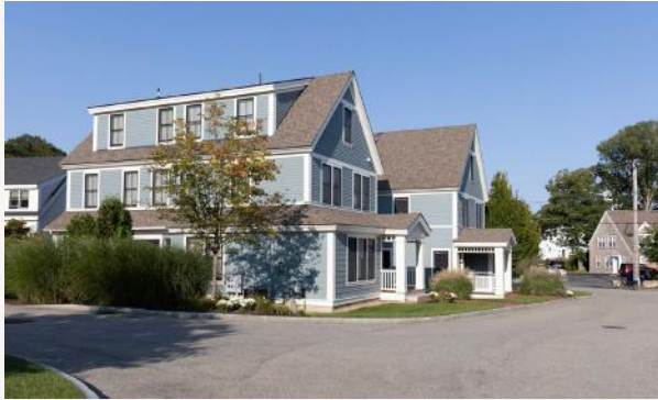
Saw Mill Circle existing conditions. Source: class photography
