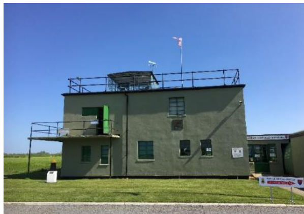
RAF Framlingham Control Tower
