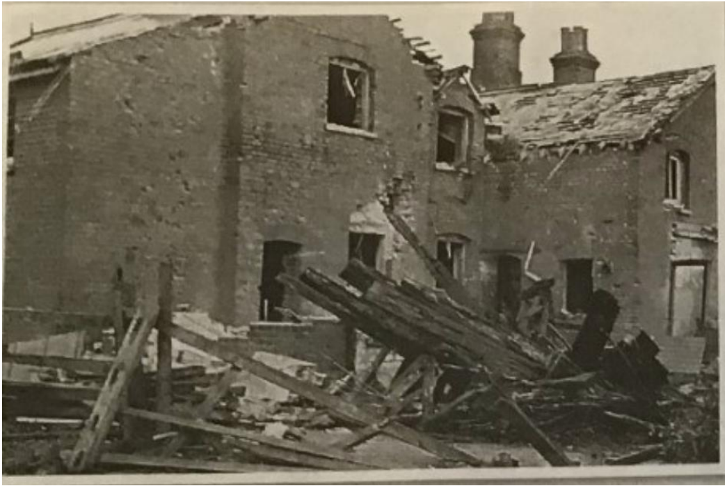
Above Railway Terrace, bombed 21st November 1940
