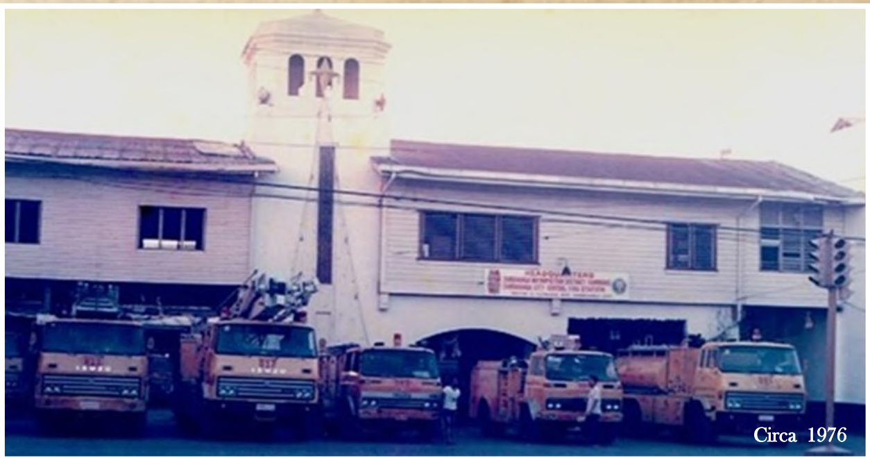
In 1976, a pivotal moment marked the history of the Fire Station Building as it welcomed its inaugural Fire Station Commander, F/Maj Dominador A Zabala. Leading a team of thirty dedicated firefighters and boasting a fleet of nine serviceable fire apparatus, this era heralded a new chapter in fire safety and emergency response.
