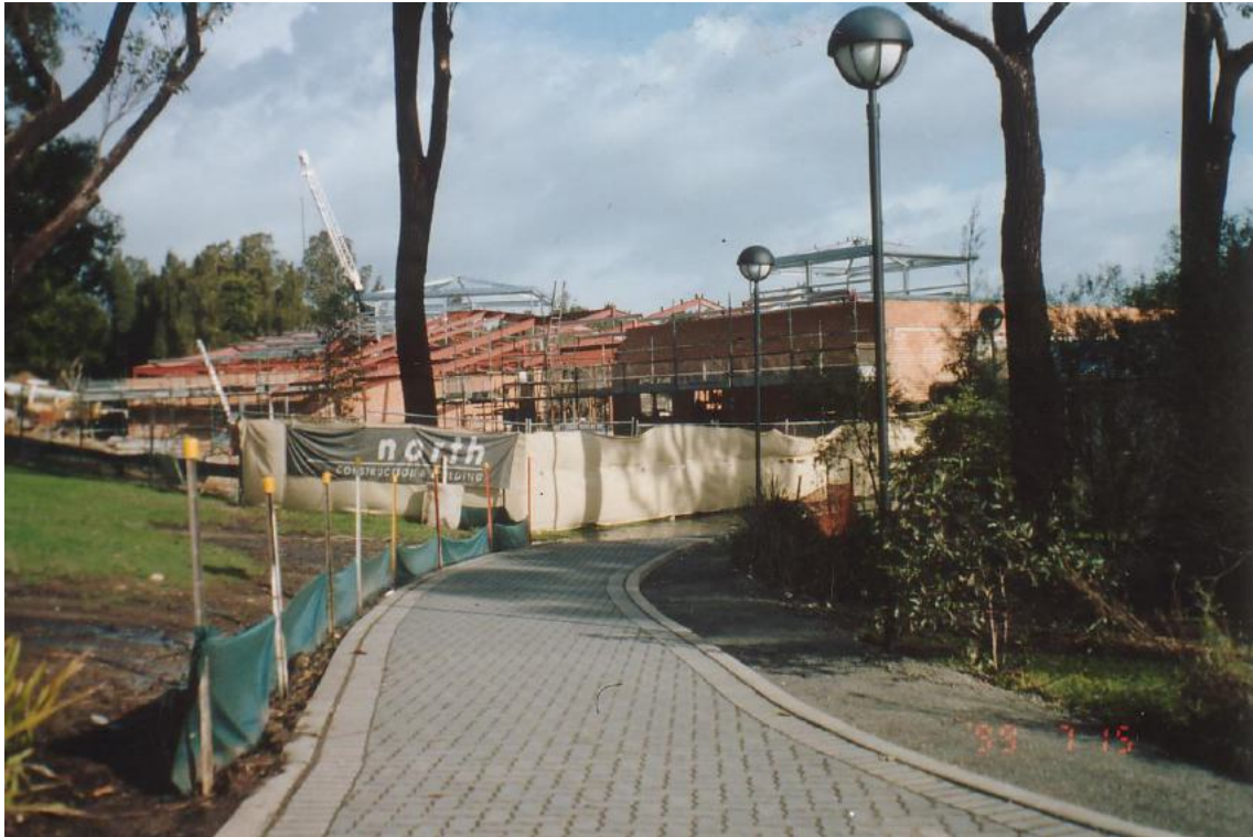
Construction of Gosford Gallery
