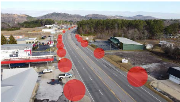
Overuse of direct access points (highlighted in red) along AL 77
