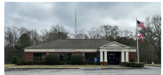
Southside Water Works offices
