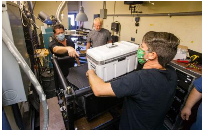
Workers install a new projector at the Keith-Albee Performing Arts Center on Tuesday, Aug. 18, 2020, in downtown Huntington.
