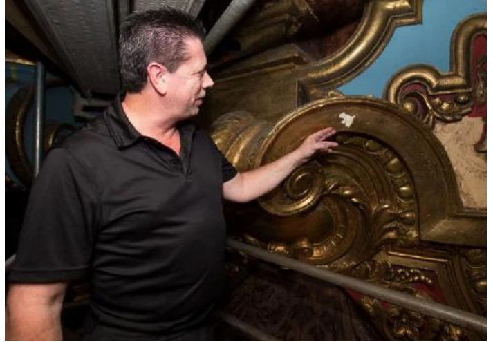
Building manager Gary Cooper points to chipped plaster being repaired by the restoration workers on Tuesday, July 9, 2024 the Keith-Albee Performing Arts Center in downtown Huntington.
