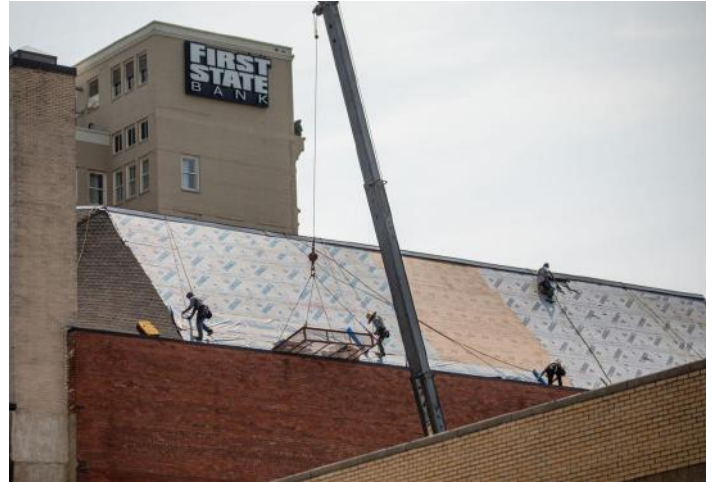
Workers complete repairs on the roof of the Keith-Albee Performing Arts Center on Tuesday, in downtown Huntington.
