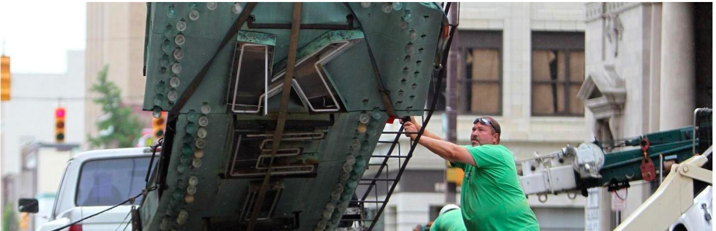
Clifton Mills and other workers from Paris Signs remove the top half of the Keith-Albee sign from the Keith-Albee Performing Arts Center building on Friday, July 8, 2011, in Huntington.
