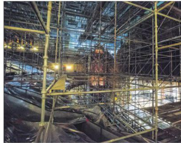
Scaffolding spans the entire theater space inside the Keith-Albee Performing Arts Center, photographed on Wednesday, May 8, 2024, in Huntington.
