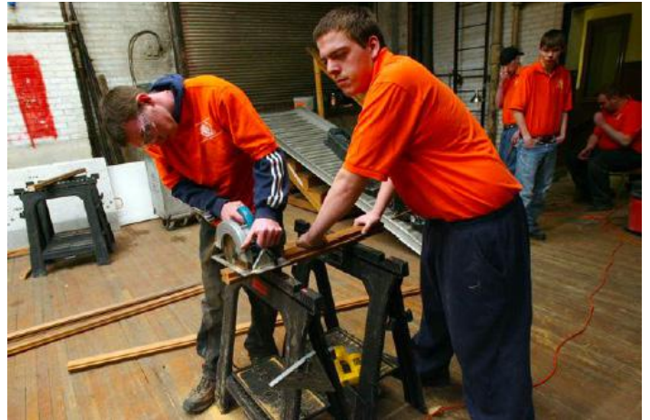
Billy McGhee, left, and Seth May cut wood as they and other students from Collins Career Center make repairs on the stage the Keith-Albee Performing Arts Center on Friday, Jan. 29, 2010, in Huntington.
