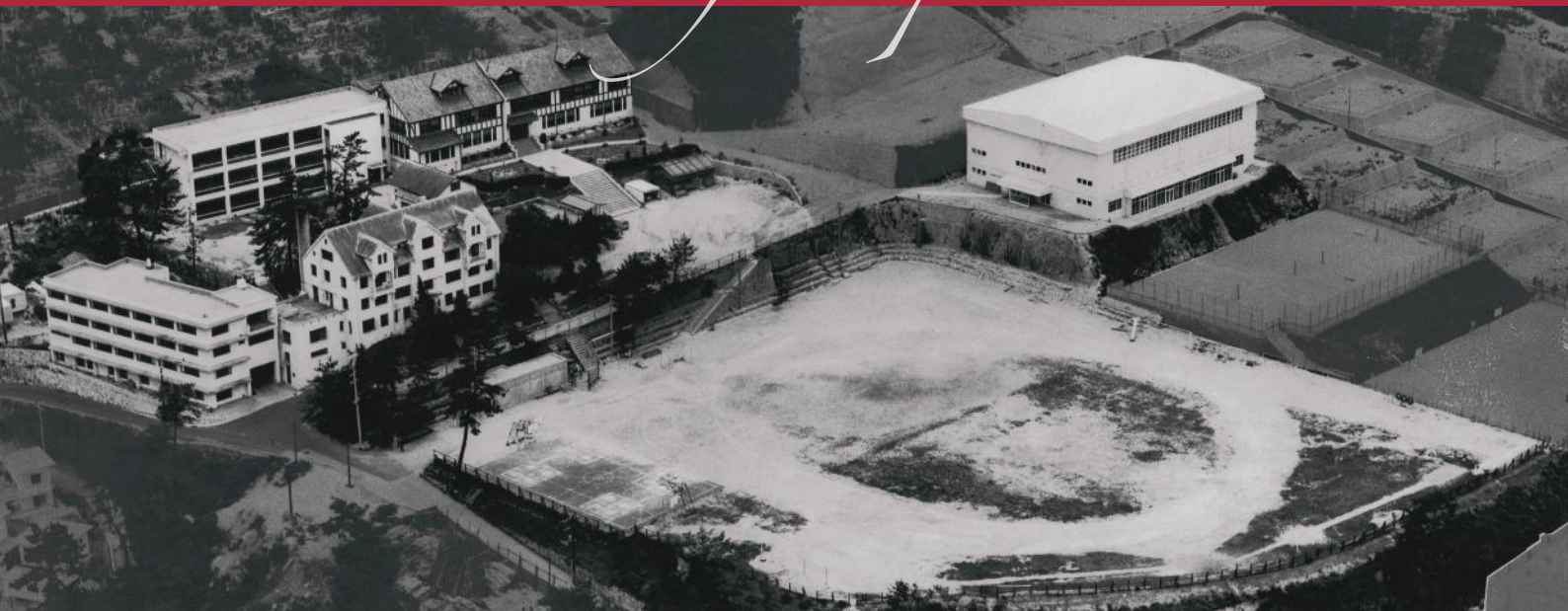
1966 Aerial view of the Canadian Academy Campus
