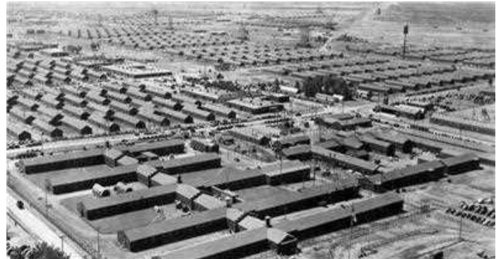
The Hanford Construction Camp housed 50,000 people at its peak.
