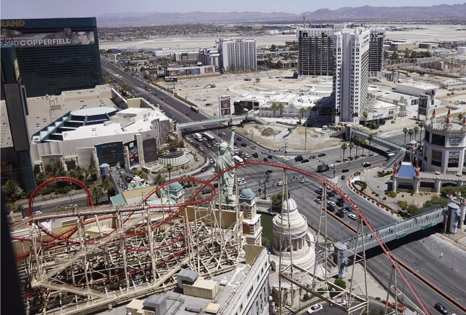
Work in progress: the site of the Tropicana casino, now under development as a ballpark for Major League Baseball's Athletics
