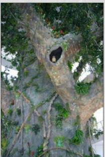
The clients' intent was to lay claim to building the largest artificial tree in the world. It is over 11 metres in diameter at the base, through which the public can walk and the diameter where it "breaks through" the ceiling is still 6 metres wide.
