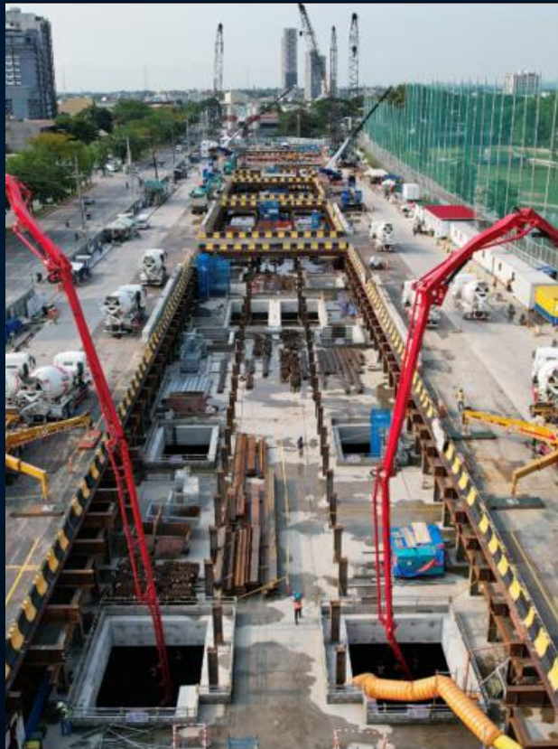
Metro Manila Subway (TBM 3 & 4) Manpower Supply
