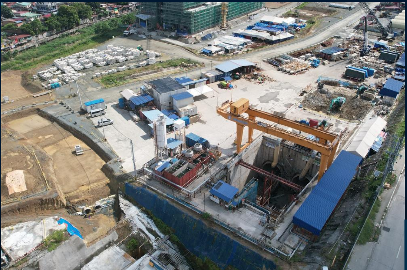
Metro Manila Subway Project - Launching Shaft Area
