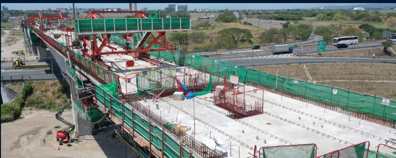
Malolos-Clark Railway Project CPN-02 – Steel Box Girder
