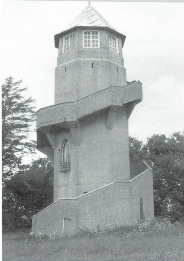
WAPPINGTHORN WATERTOWER FAR RIGHT: SHAM RUINED CHURCH IN MILTON ABBAS
