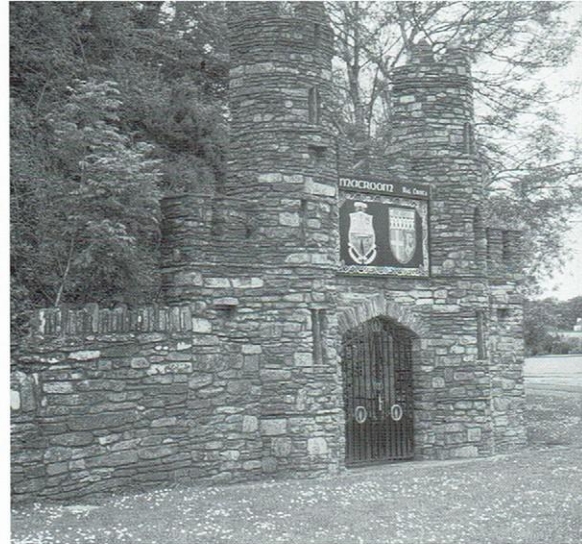
TOP: SHAM TOWNGATE, MACROOM BELOW: REBUILT COTTAGE ORNÉ, KILFANE
