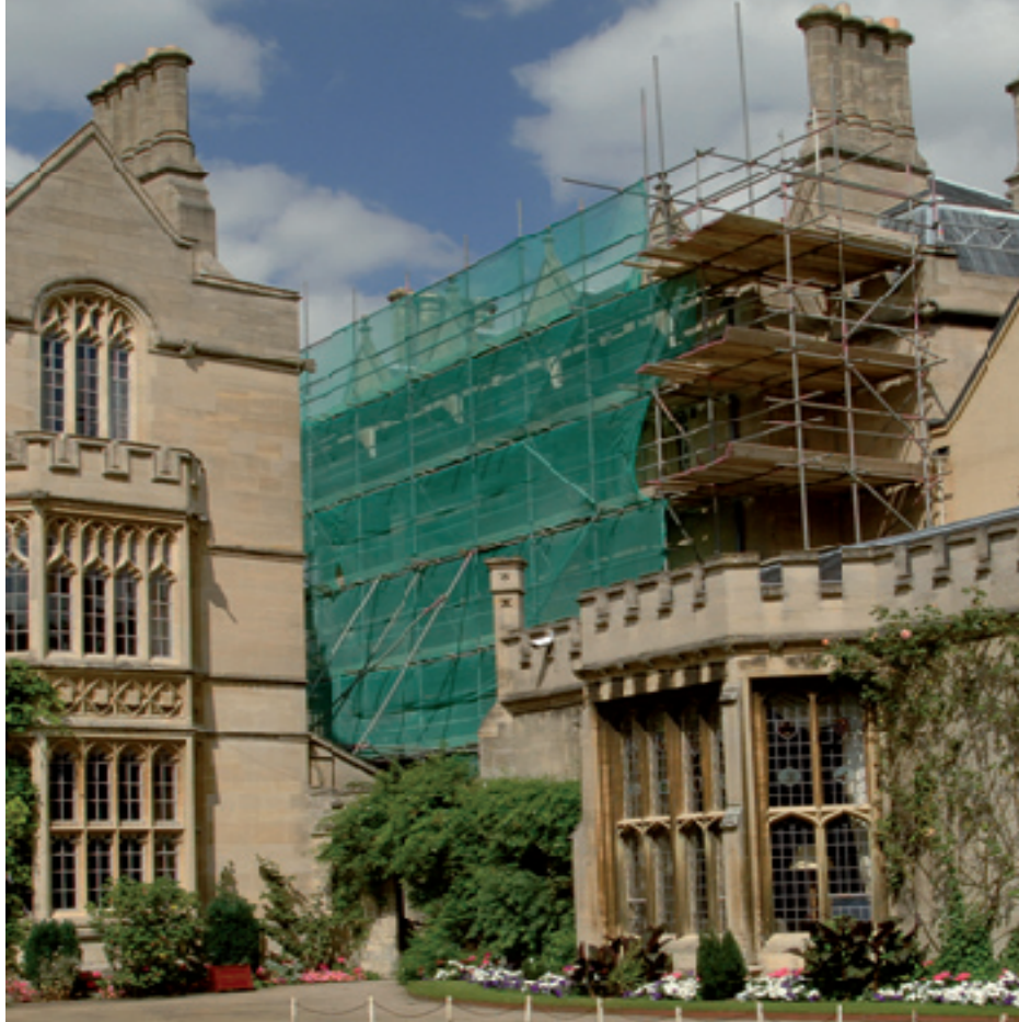
Staircase 8 in scaffolding from the Chapel Quad, July 2005
