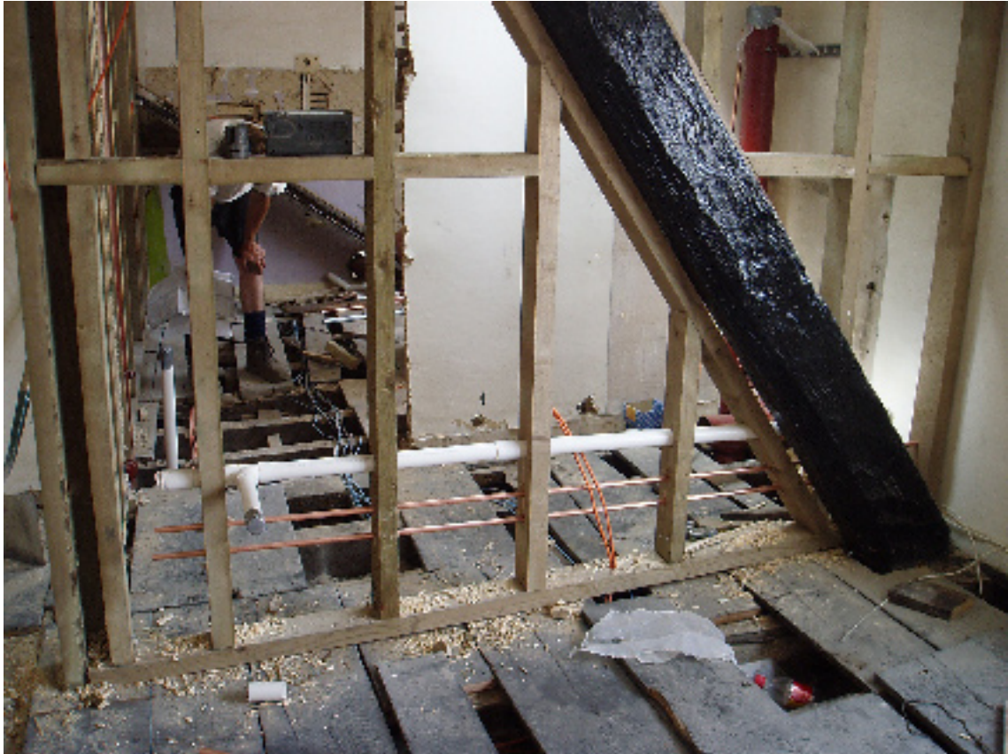
Renovation in progress on Staircase 18
