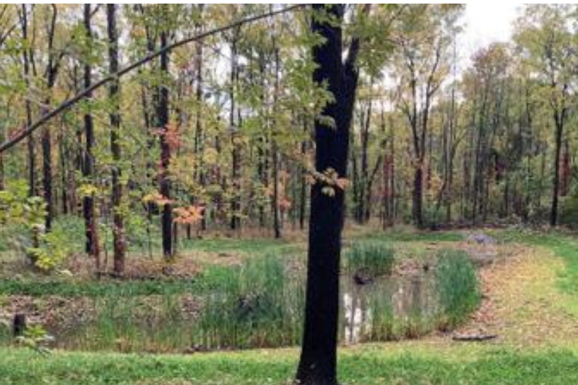
The 20-acre project area on the FLCC Campus now provides an additional 20 million gallons of stormwater storage, keeping pollutants and sediment out of the lake
