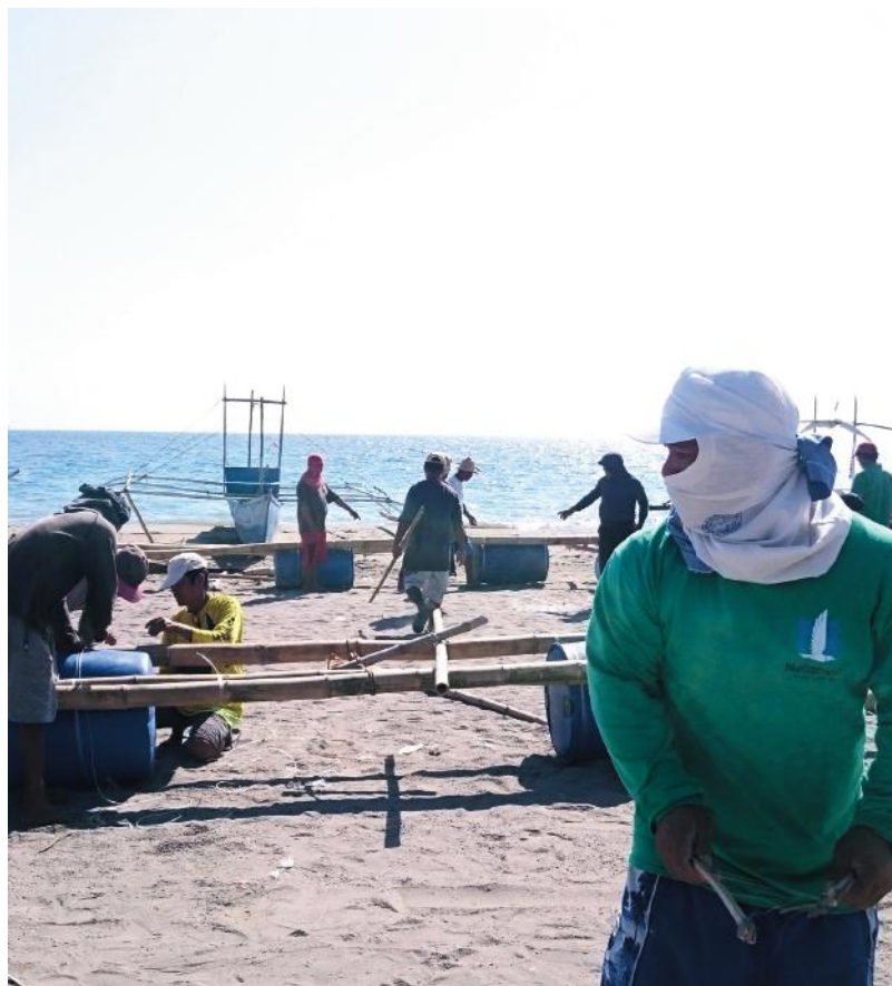
(Top) Construction of 10x10 meter fish cages through distributed fish cage materials in Sta. Cruz, Occidental Mindoro.
