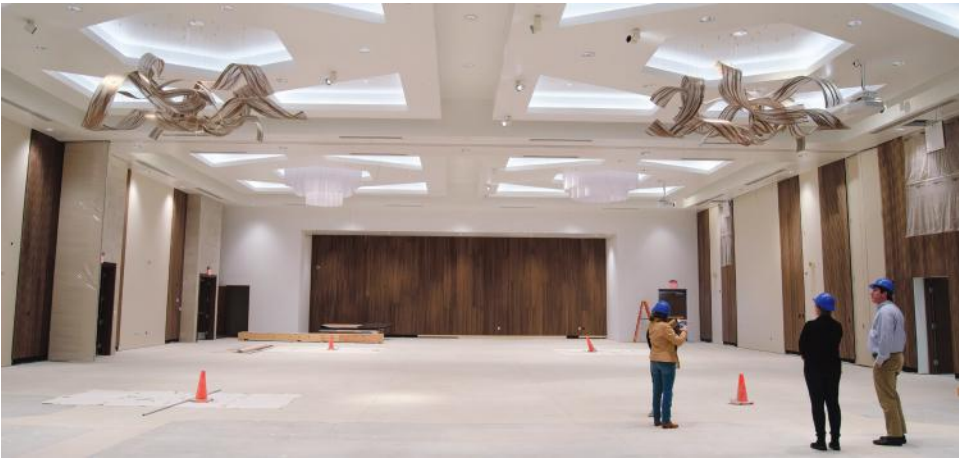
Kaplan Community Hall inside The Ora nears completion
