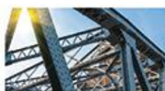
steel structure construction
