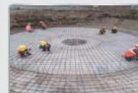
SEWERAGE PIPELINE & TREATMENT PLANT AT BARWANI & SENDWA DISTRICT, MADHYA PRADESH
