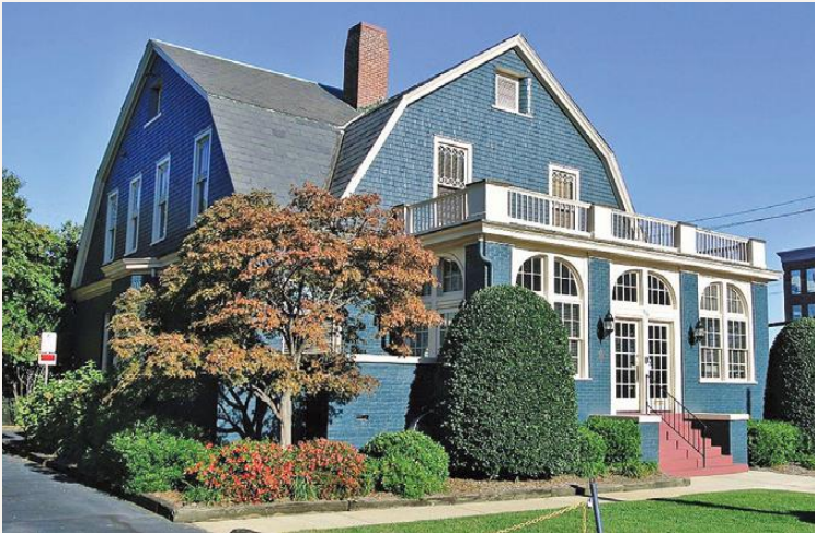
John and Idella Mayes House , Charlotte. 1902. The only surviving turn-of-the-century house in Charlotte's old Second Ward, and one of the few remaining houses along once-fashionable Morehead Street. Photos show its condition in the mid-1970s and in 2020; at both times the house was imminently threatened. Easement Donor: Morehead Street Properties LLC (structured by GBX Group, Cleveland OH).
