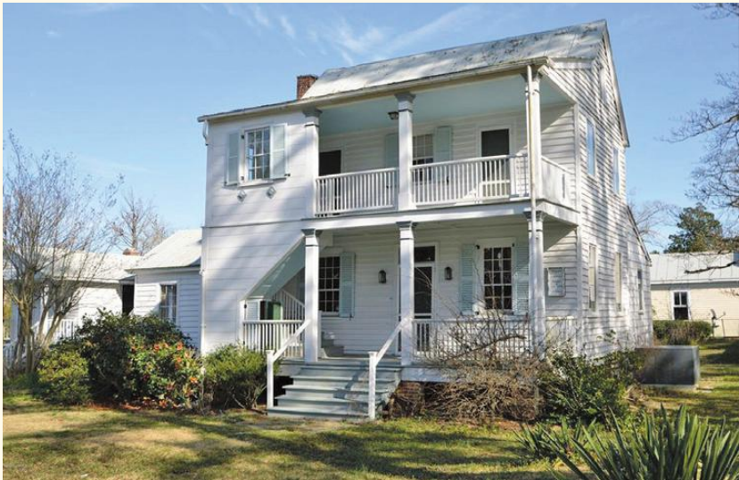
Bryan Lavender House , Pollocksville, Jones County. c. 1825. Of particular architectural interest due to its double-tier front porch with an enclosed end and exterior stair. Donated by John Fox and Libby Heisman, Star Tannery VA. Buyers: Janet and Larry Parson, Kinston.
