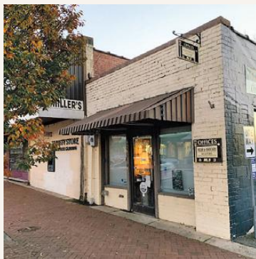
622, 626 (pictured) and 632 N. Trade Street, Winston-Salem. 1920s. Commercial buildings that supported the everyday lives of tobacco farmers and workers in the nearby factories and warehouses. Easement Donor: Trade Street Properties, LLC (structured by GBX Group, Cleveland OH).
