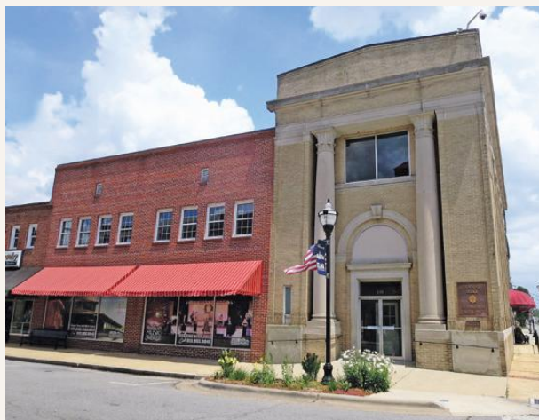
Former Selma Town Hall, Selma, Johnston County. 1920-1950. Several historic buildings, including the historic 1922 People's Bank, linked together for a single user. Buyer: B2B Selma LLC, Raleigh.
