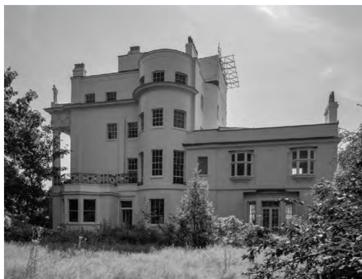
EXISTING NORTH-WEST FACADE (Photograph)
