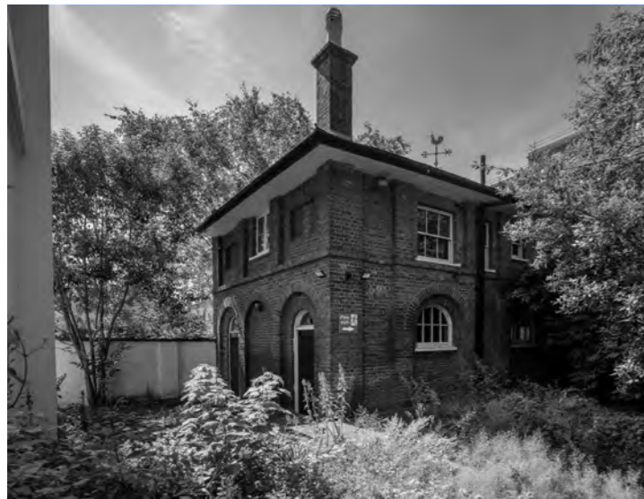
EXISTING STABLE BLOCK (Photograph)
