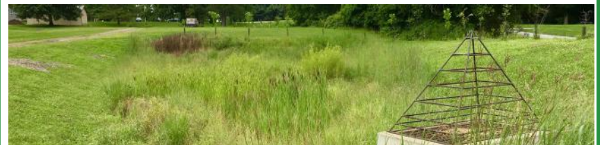
Bioretention Basin | Source: Hillendale Elementary School
