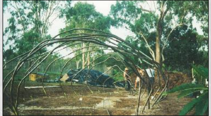
Creating the Armature - additional framing added
