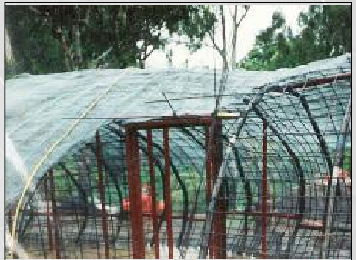
Adding the door frames & application of wire netting over 10mm mild steel bar armature. (It is built in concrete)
