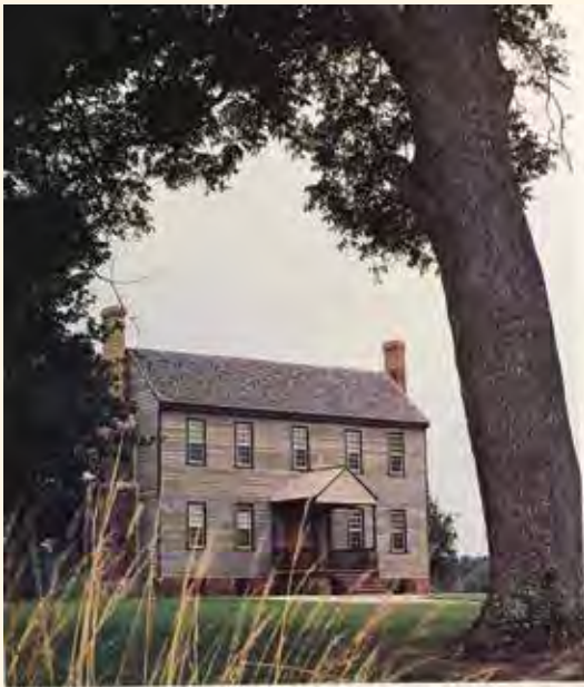
With additions removed, the 18th-century plantation house returns to its original form. Staining rather than painting makes it look weathered.
