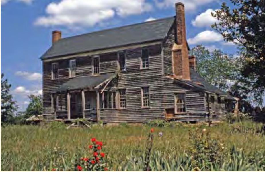
Before restoration, Patty Person Taylor House, Franklin County, 1980.
