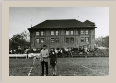
• LOOKING NORTH MASON GYM •
