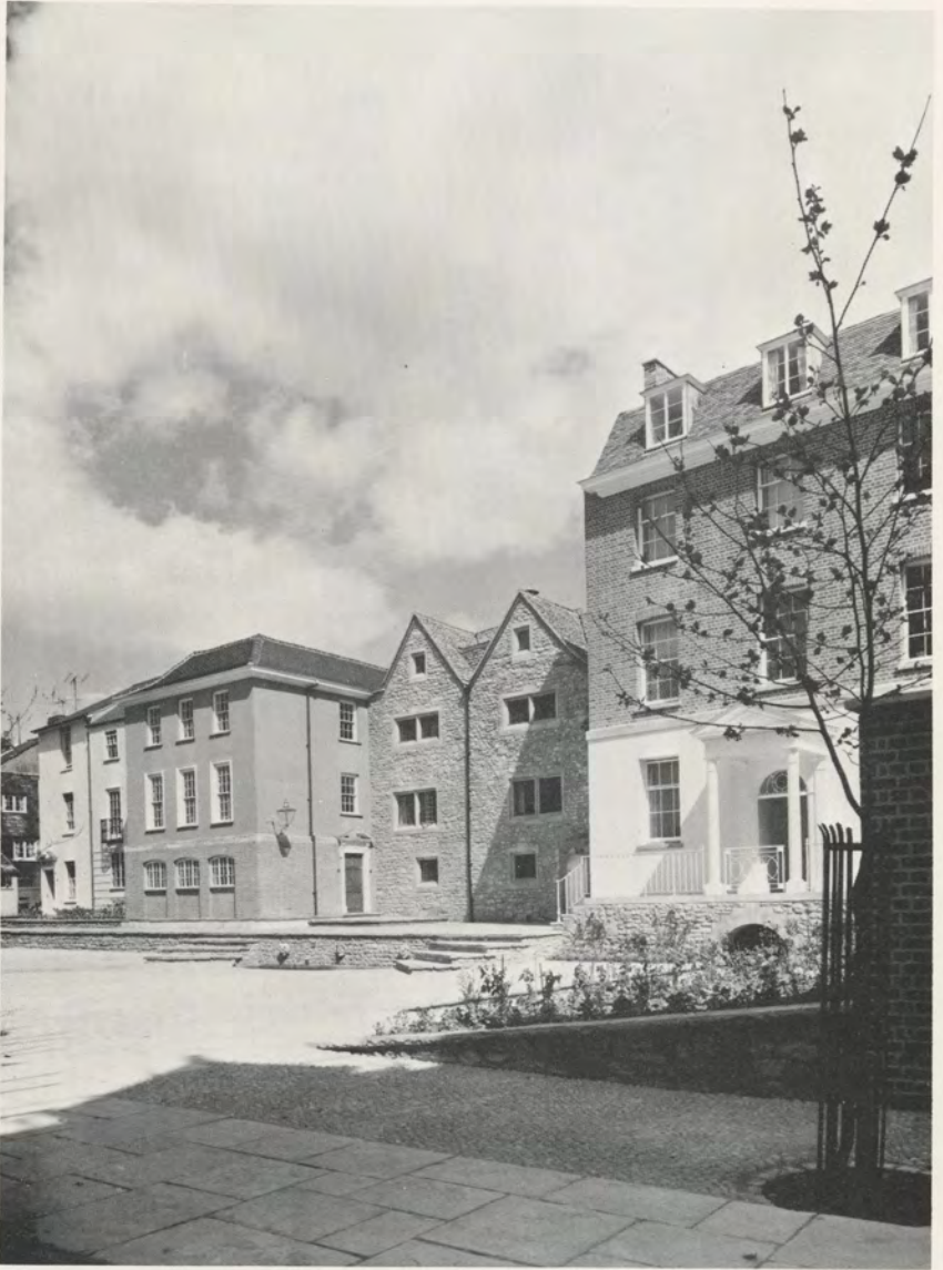
The restored elevation of the Quadrangle looking from the South East.
