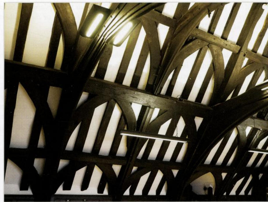
(8) The Carow-Coke roof of the Almshouse 'Great Attic', c.1529. Probably built as a decorative roof above a first floor hall.
